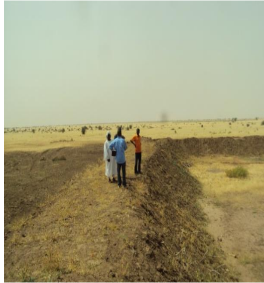
Plate (G): Earth Embankment at Sarafaya
